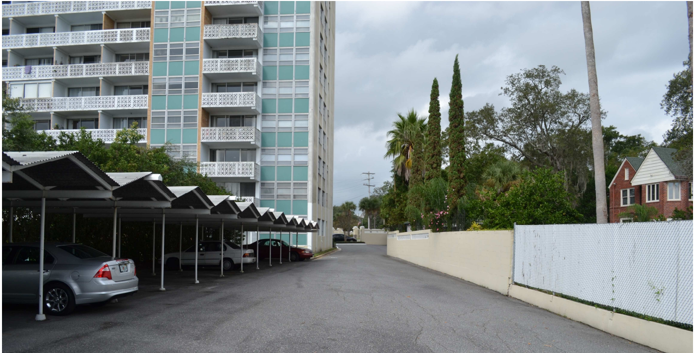
The existing area of the site between the Commander Apts. and the single-family residences to the northeast on DuPont Cir.; facing northwest towards St. Johns Avenue
